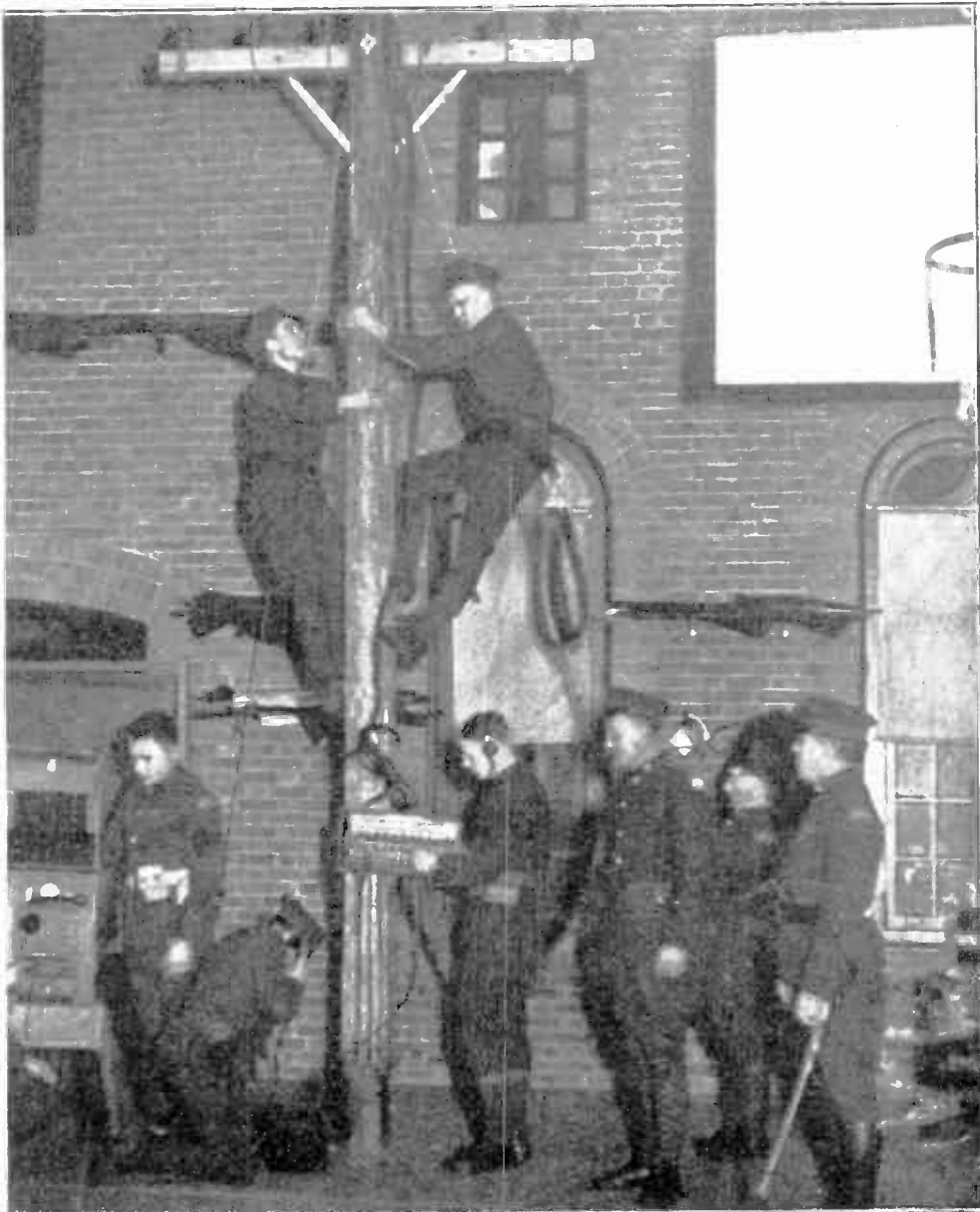
Company B, 101st Signal Battalion, N. Y. N. G., are keeping abreast of the times in modern operation. In emergency they utilize telephone and telegaph wires for both wire and excellent instruction is given to members of the signal division in the National Guard. They are shown tapping a telephone line.
